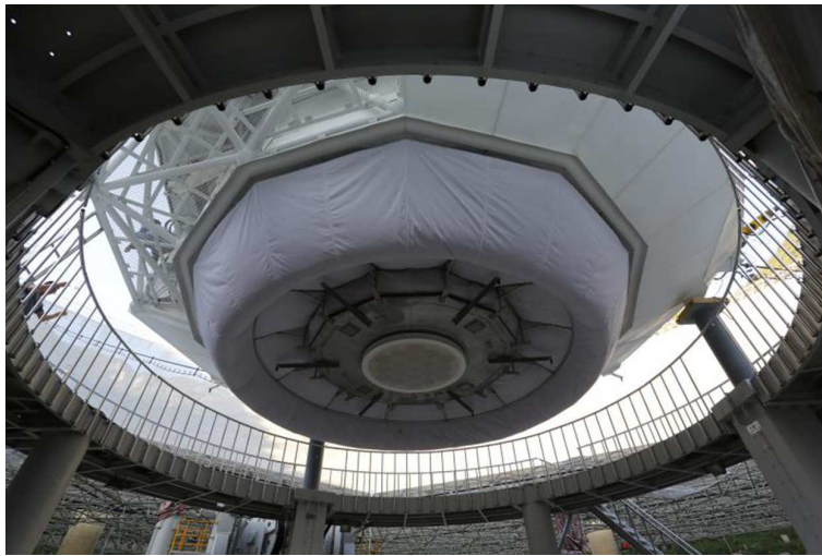
Fig. 4 Combined shielding measures for the feed cabin.
